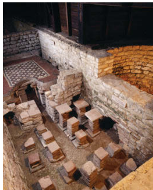
Source 4.33 The remains of a mosaic floor and hypocaust from Chedworth Roman villa. The tiles supporting the floor and the hole to the furnace can be seen.
