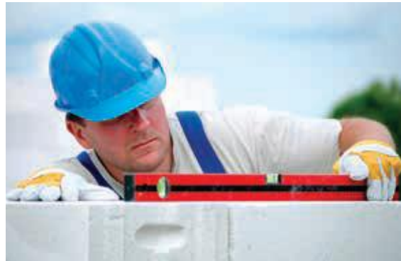
A builder uses a spirit level to check that bricks are horizontal
