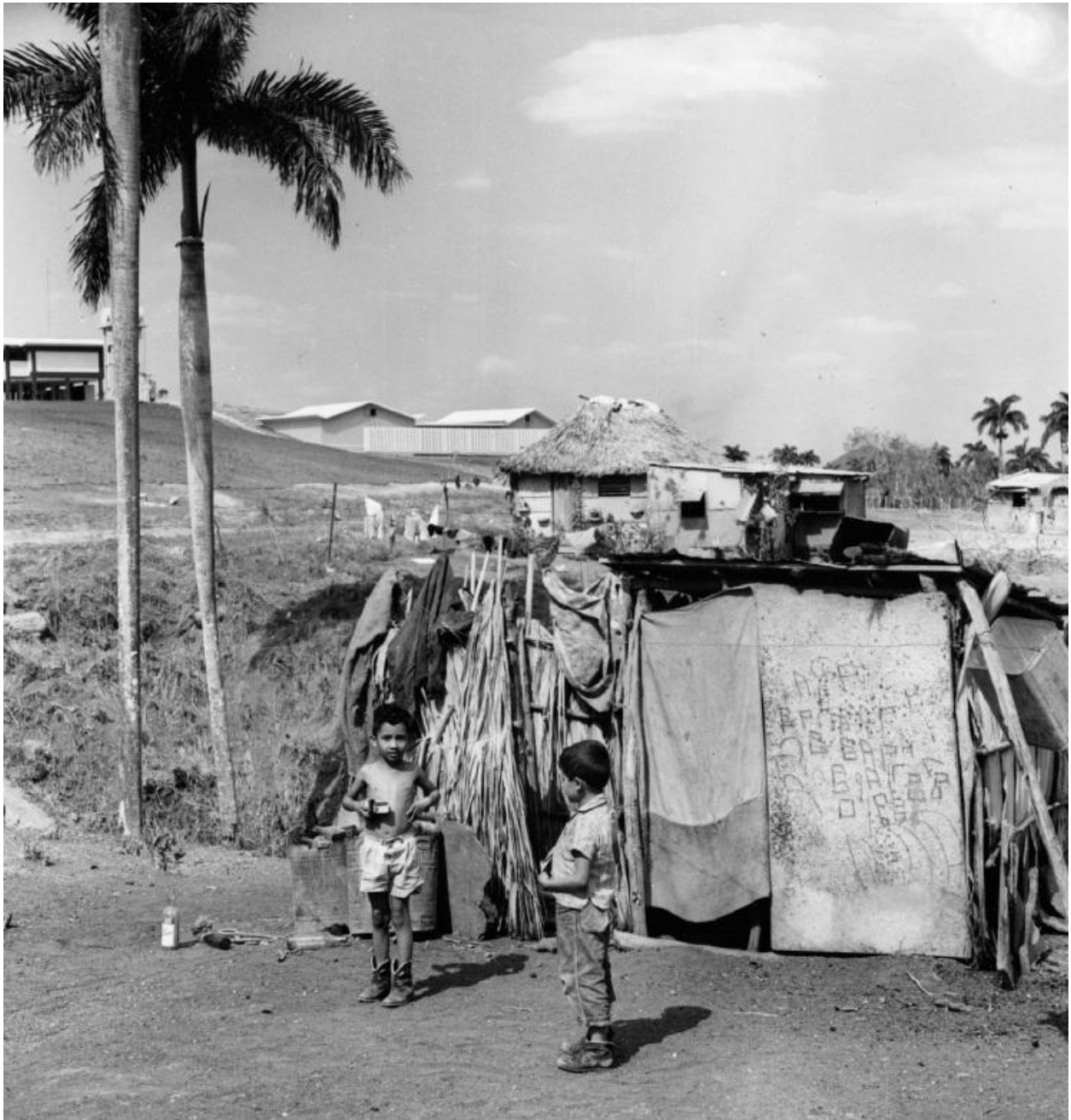
Figure 5.9 Poor peasant housing in Oriente Province, Cuba, before 1959
