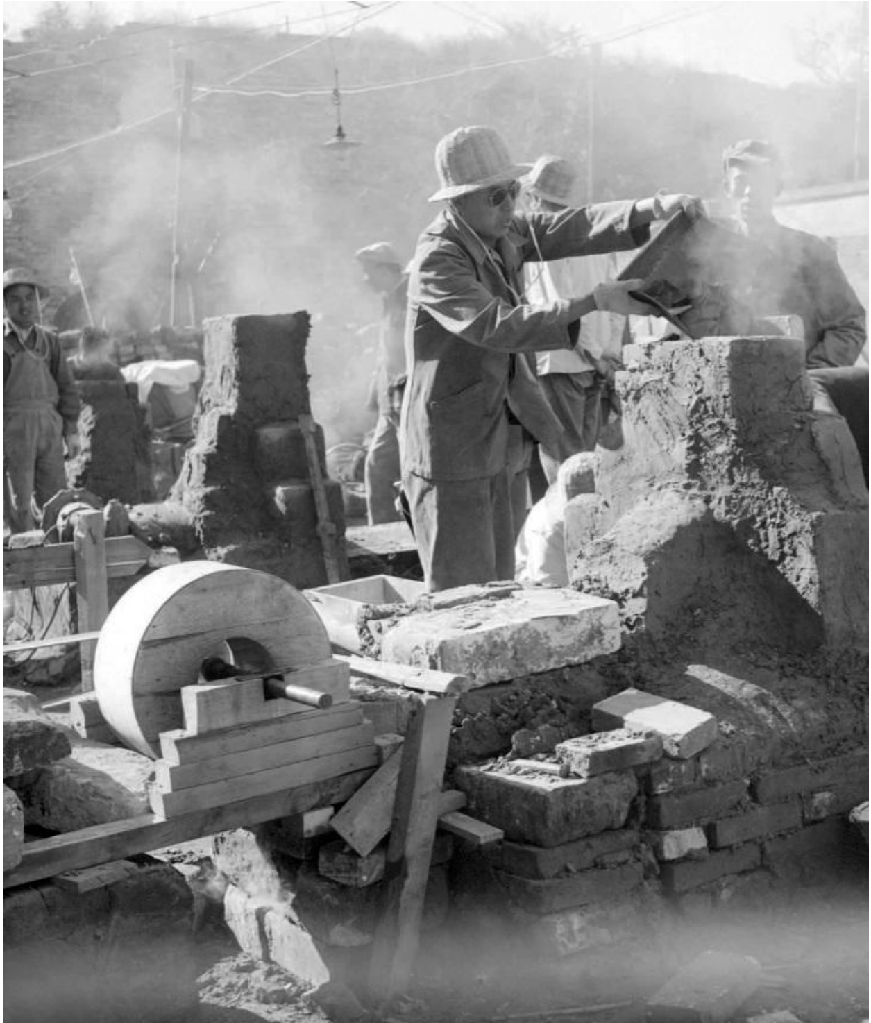
Figure 4.13 Backyard furnace construction in Beijing during the Great Leap Forward, October 1958
