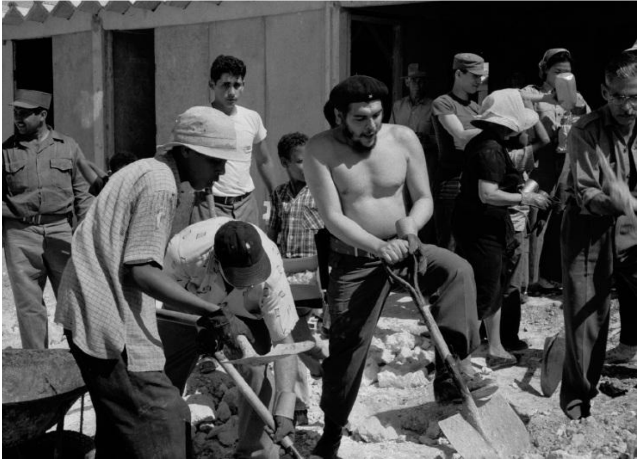
Figure 5.19 Guevara, minister of industries, taking part in voluntary labour at a public housing construction project in Havana in 1961; he gave most of his spare time to such activities
