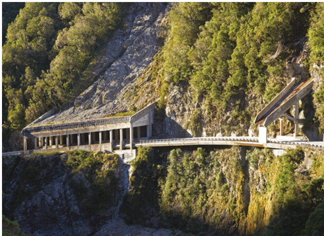
Source 6.12.3 Avalanche bridges are used to protect vital transport infrastructure.
