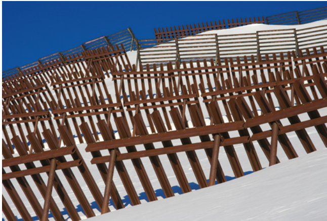
Source 6.12.2 Snow racks are used to retain snow, thereby reducing the risk of avalanches.
