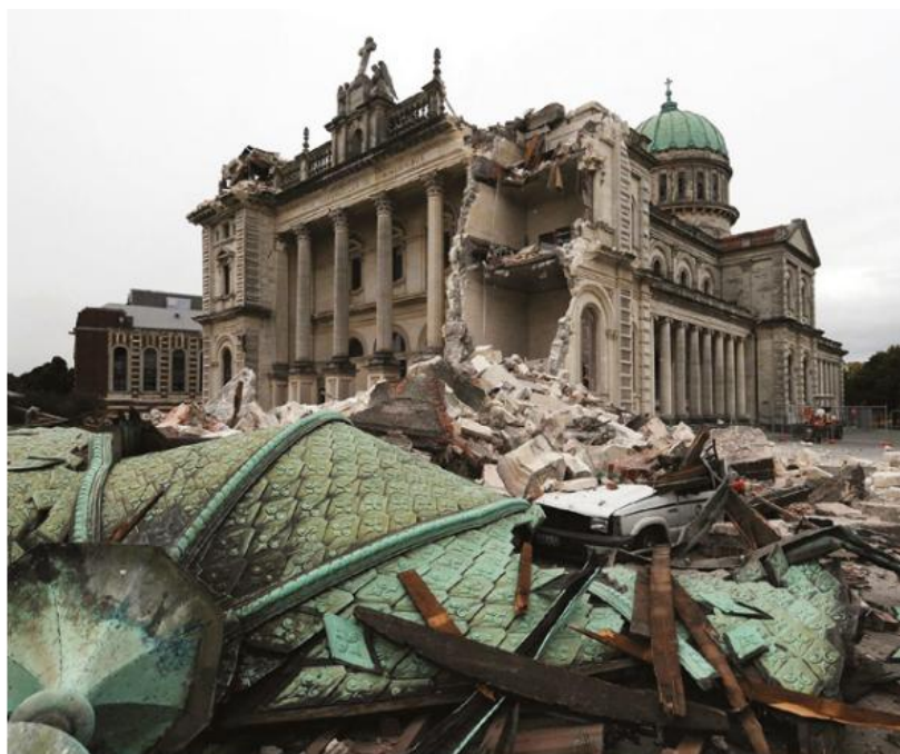
Source 6.7.3 The primary devastation caused by the 2010 earthquake in Christchurch, New Zealand
