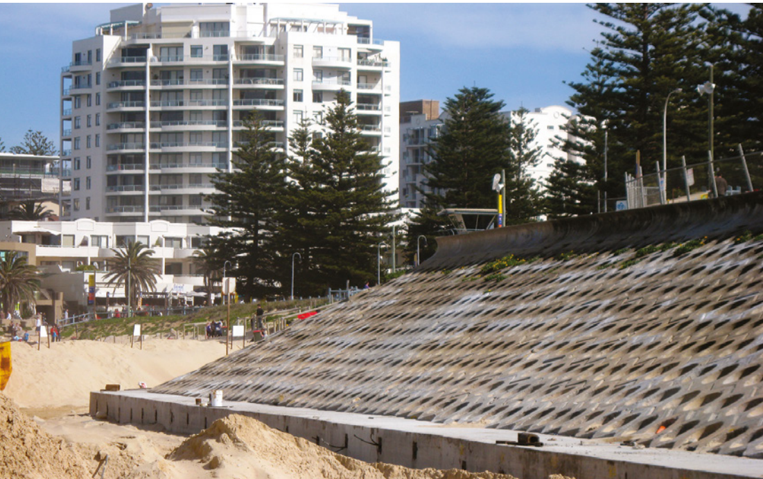
Source 7.4.6 Sea walls are examples of 'hard engineering' used to protect coastal development. While such walls absorb the power of the waves, they are expensive to build and maintain, and can cause more erosion because they reflect much of the energy of the waves; that is, as the wave bounces off the wall it carries away with it sand from the beach.
