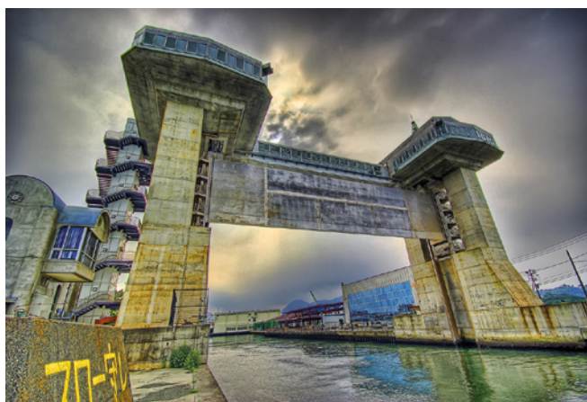
Source 6.13.2 A tsunami barrier and gate, Numazu, Japan
