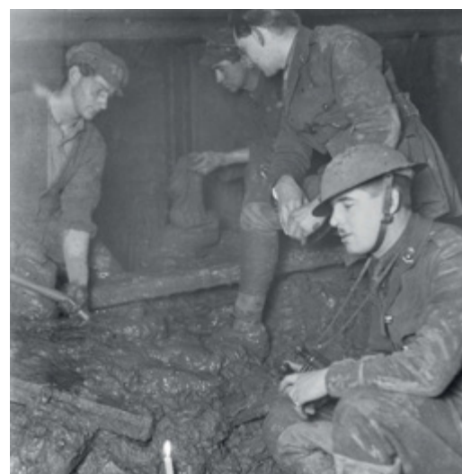
Source 6.41 A photograph taken on 22 January 1918 shows members of a British Tunnelling Company attached to the Australian Corps making a dugout in the slimy mud beneath an artillery observation post near Messines, in Belgium.
