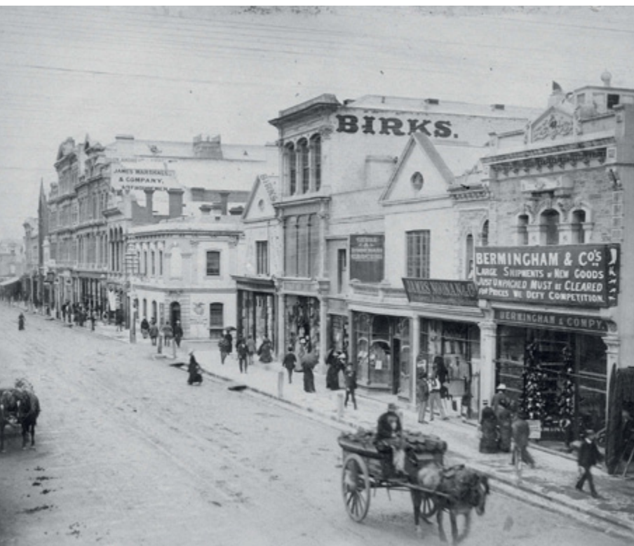
Source 4.18 Rundle Street, Adelaide, c. 1865
