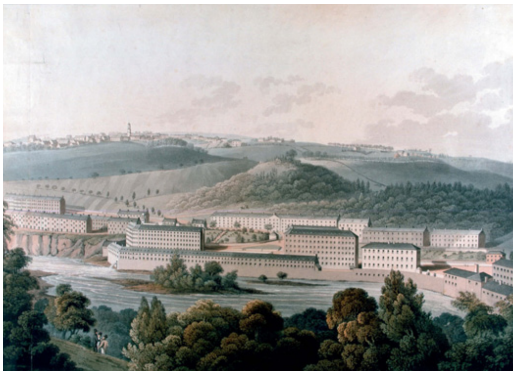
Source 1.40 An artist's impression of Robert Owen's cotton mill at New Lanark in 1818. Note the fast-flowing river in the foreground that was used to power the mill.
