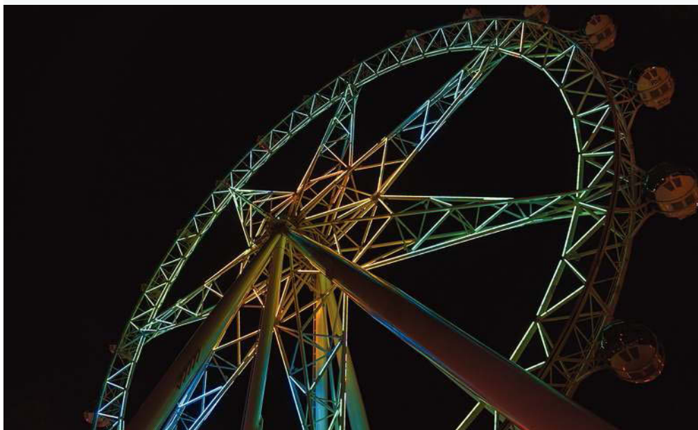
FIGURE 4.1 Decorative lights that are connected in series, such as those on the Melbourne Star Observation Wheel, can contain shunts which allow the circuit to remain closed if the filament breaks.
