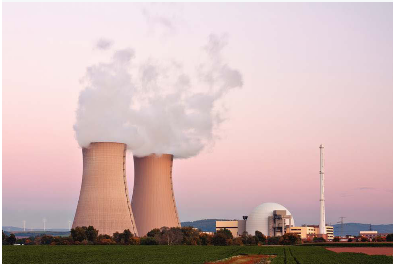
FIGURE 8.1 Nuclear power plants use nuclear fission to create roughly 13% of the world's electricity supply.
