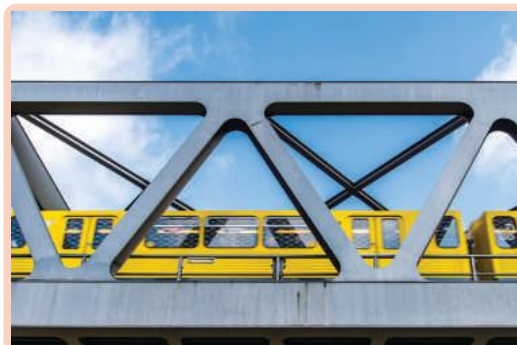
The triangular shapes in this bridge in Berlin help distribute weight evenly and provide rigidity, making the structure strong and stable.
