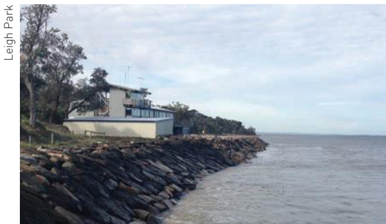
Protective sea walls constructed in front of the Yacht Club on Somers Beach, Victoria
