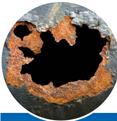
Figure 5.9 Rust will 'eat away' iron metal and cause the formation of holes. When iron reacts with the air and the moisture, it forms a completely new substance that can be washed or scraped away.
