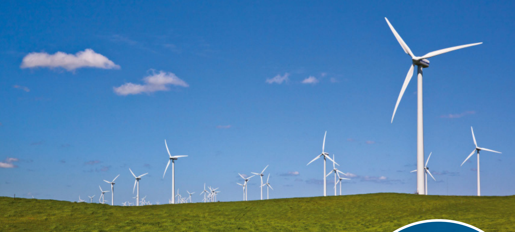
Figure 3.61 A wind farm in South Australia.
