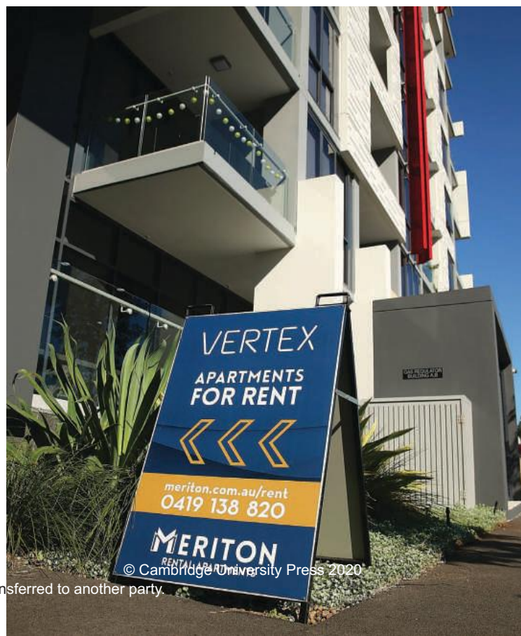
Figure 14.11 Landlords have an obligation to ensure premises are habitable, clean, safe and secure.
