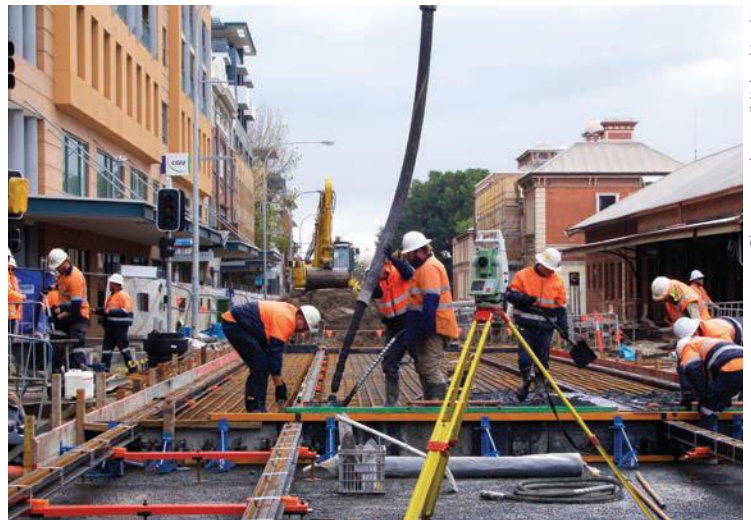
FIGURE 3.2.1 Construction workers laying the rails for the Newcastle light rail. Wages are paid to employees who work for an hourly rate of pay.
