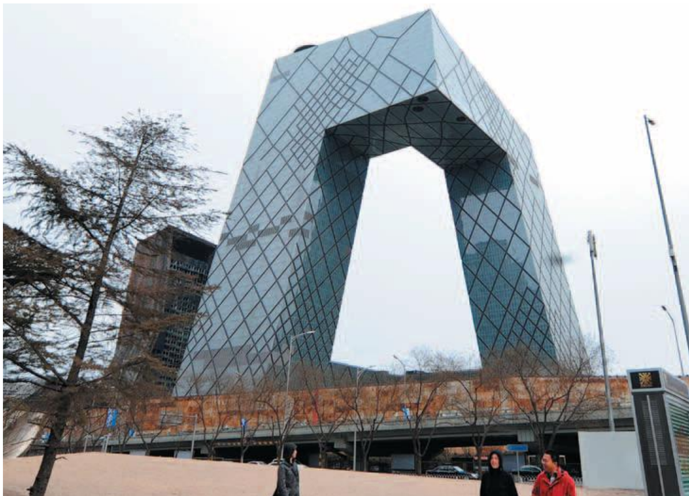
CCTV Building and the Television Cultural Centre (TVCC), Beijing, China, 2008 Photo: Frederic J. Brown AFP/Getty Images
