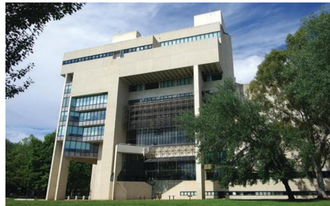
FIGURE 10.9 High Court of Australia, Canberra
