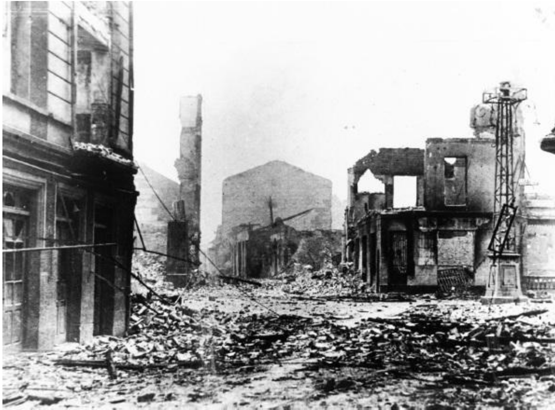
Figure 3.12 Bomb-damaged buildings in Guernica after the city was devastated by the worst air raid of the Spanish Civil War in April 1937
