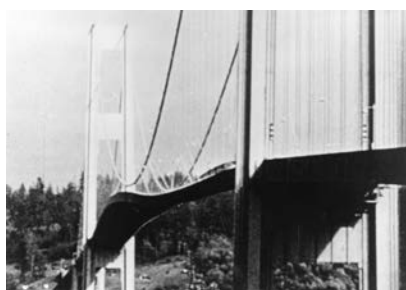
Figure 15.19: The Tacoma Narrows Bridge in Washington State in the United States oscillating before collapsing in 1940, a victim of resonance.
