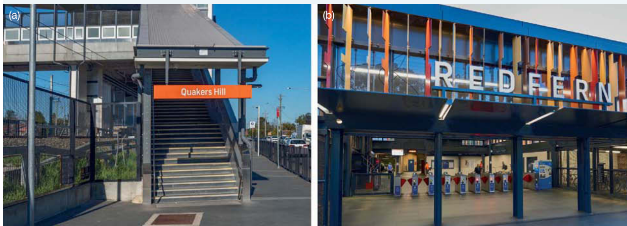
FIGURE 5 (a) Quakers Hill and (b) Redfern Metro stations, Sydney
