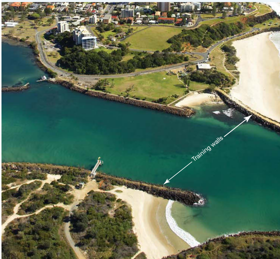
FIGURE 1 The Tweed River training walls
