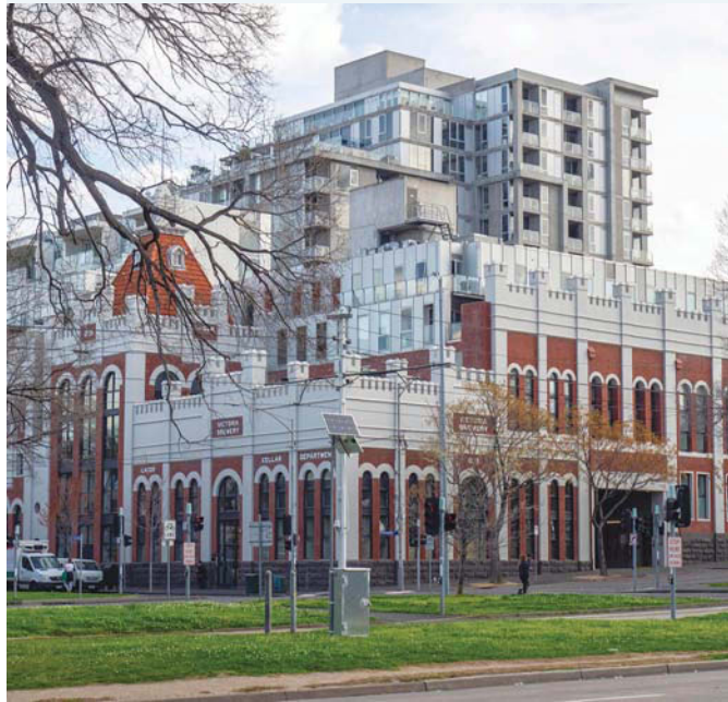
FIGURE 3 A former brewery transformed into a high-density apartment complex in inner-city East Melbourne
