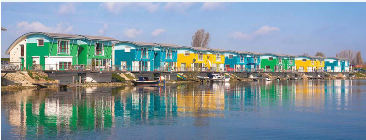
FIGURE 1 Floating houses anchored to the embankments along the waterfront at Maasbommel, the Netherlands
