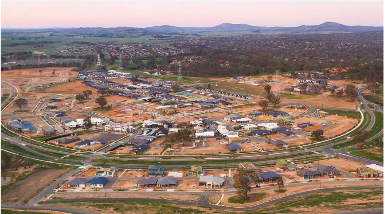
FIGURE 4 Land clearing for a housing development at Strathnairn, a new suburb in the north of Canberra
