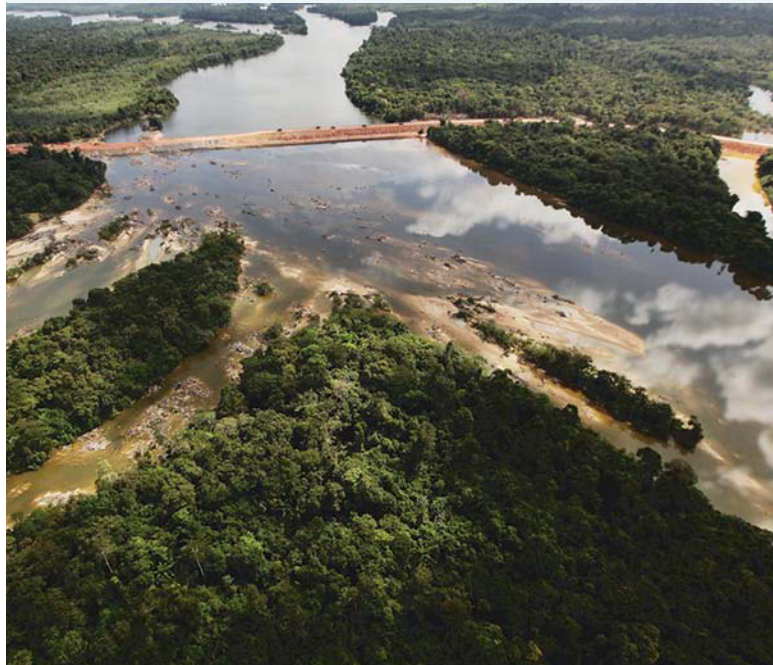
FIGURE 8 First stages of the construction of the Belo Monte Dam
