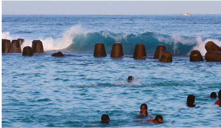
FIGURE 5 A tsunami break wall in Malé, part of the island's defenses against future natural disasters
