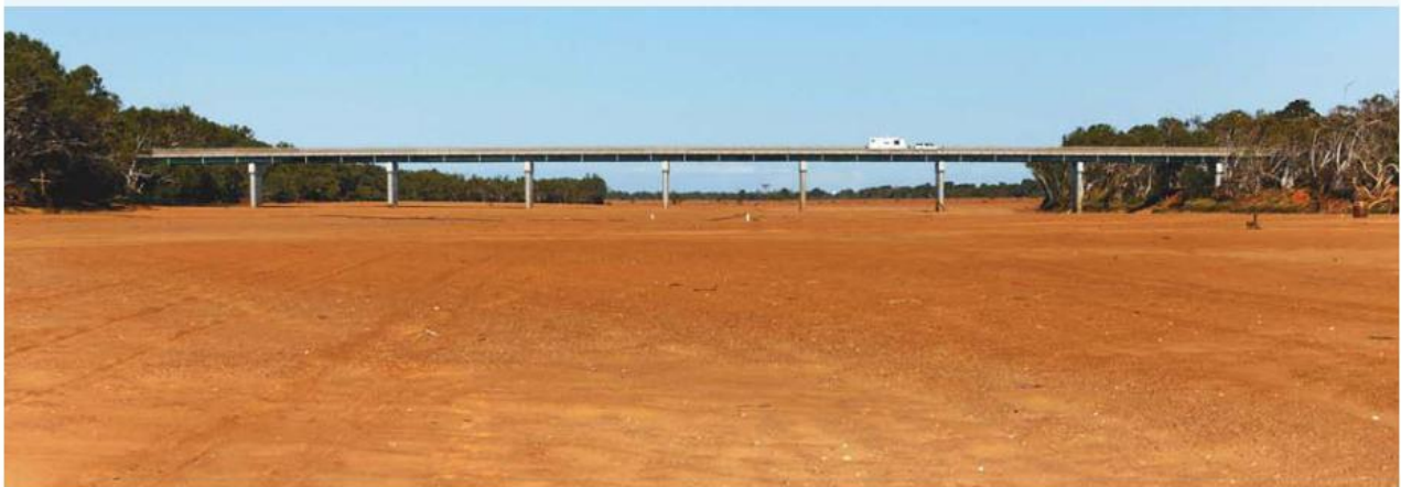
FIGURE 1 Road bridge crossing the dry Gascoyne River, Carnarvon, Western Australia
