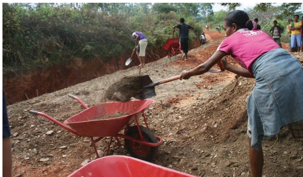
Figure 11.23 Women from a local village in Timor-Leste working on a Roads 4 Development project
