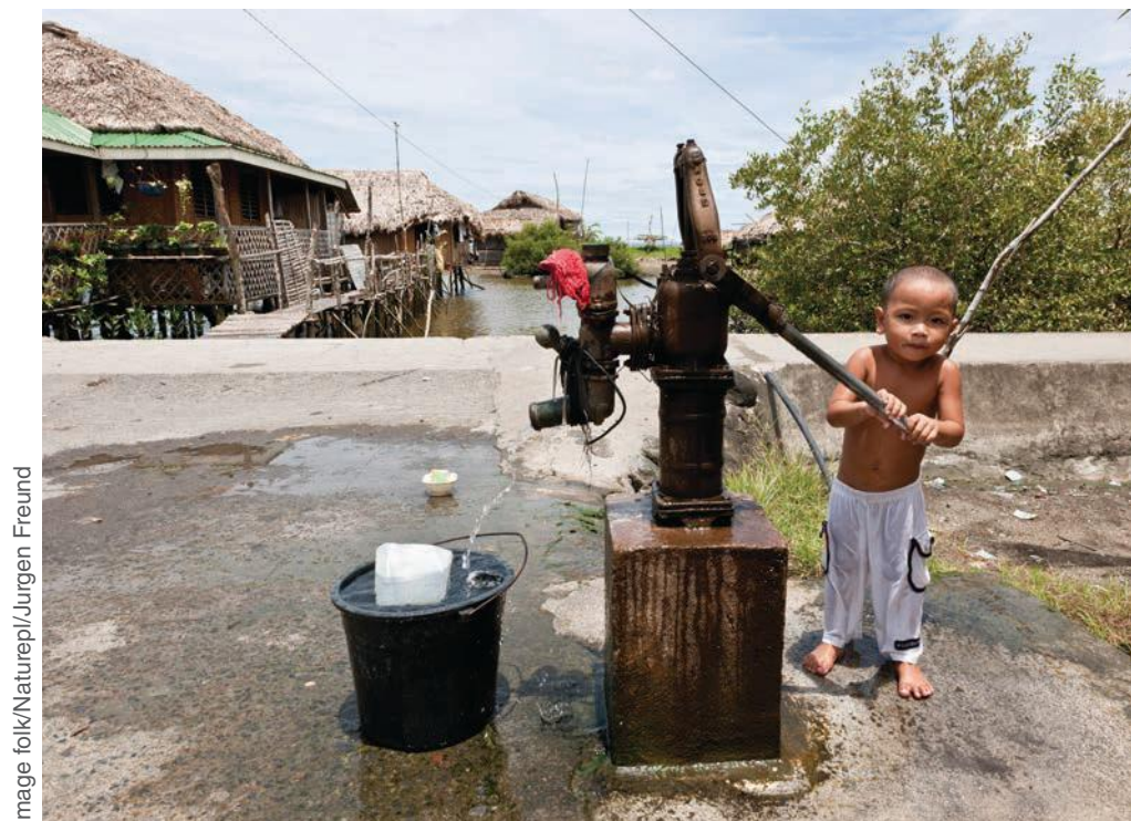
Figure 12.12 A water pump can meet the clean water needs of a community.
