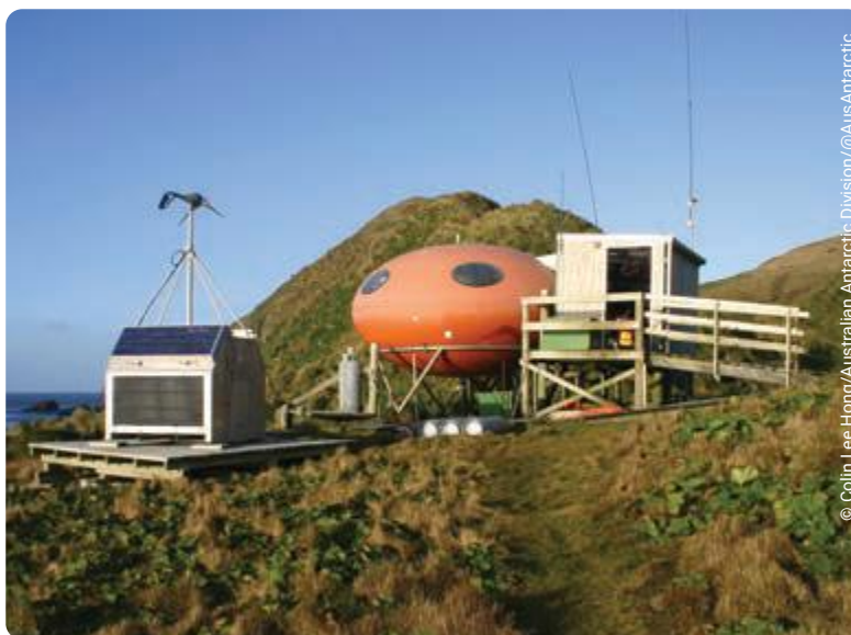
▲ FIGURE 8.6.1 A hybrid RAPS. It uses energy from wind and moving water to turn generators that produce electric power, as well as solar-powered photovoltaic cells. The back-up is a motor generator powered by fossil fuel.
