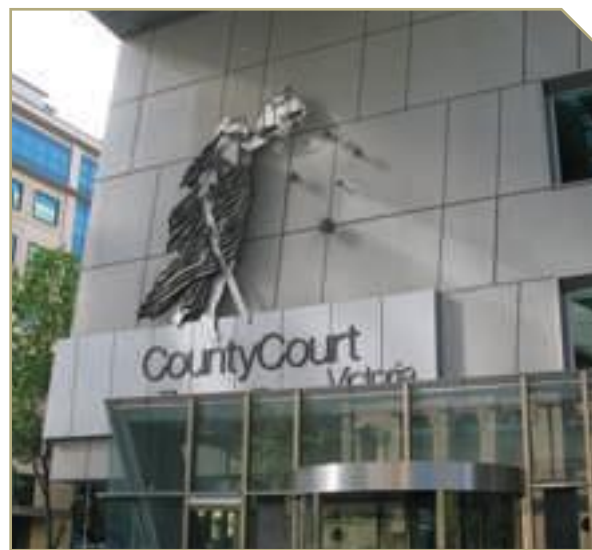
Figure 10.1.3 Victorian County Court
