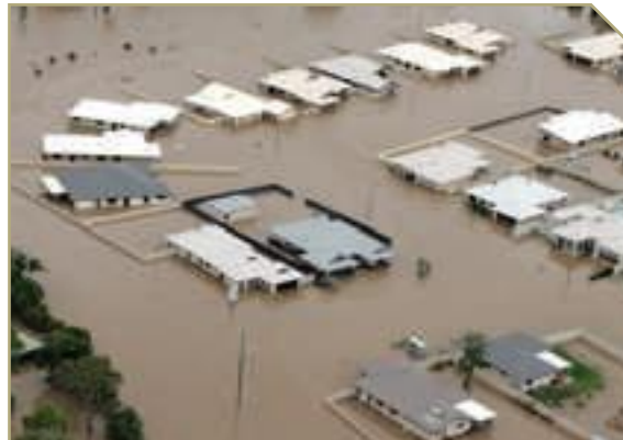
Figure 2.1.7 The federal government introduced a 12-month flood levy to pay for some of the flood damage to infrastructure in Queensland and Victoria in 2011.
