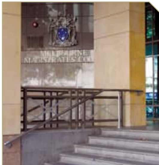
Figure 10.1.2 The Melbourne Magistrates' Court in William Street
