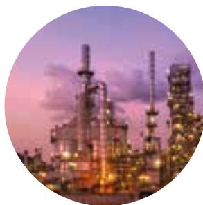
Figure 2 In oil refineries, distillation towers are used to isolate the different liquid fractions in crude oil as part of the process of making petroleum.
