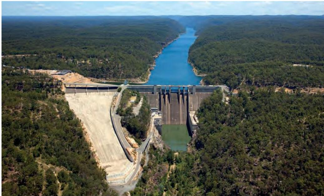
5.7 Woronora Dam, Sydney. The concrete barrier of the dam has been built across the river to impound its water.
