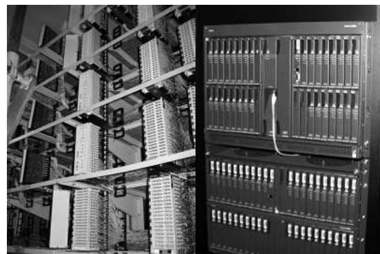
Fig 8.34 A splitter (left) and DSLAM (right).
